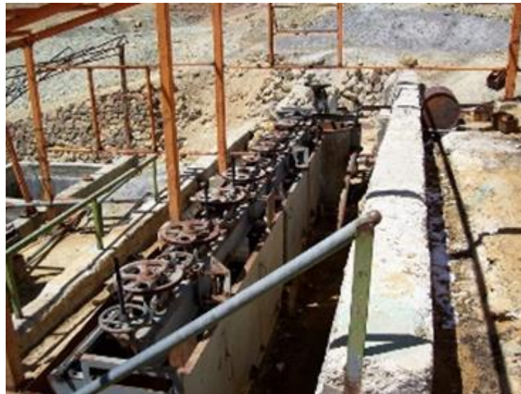
Figure 6-1: Part of the Old Flotation Circuit
